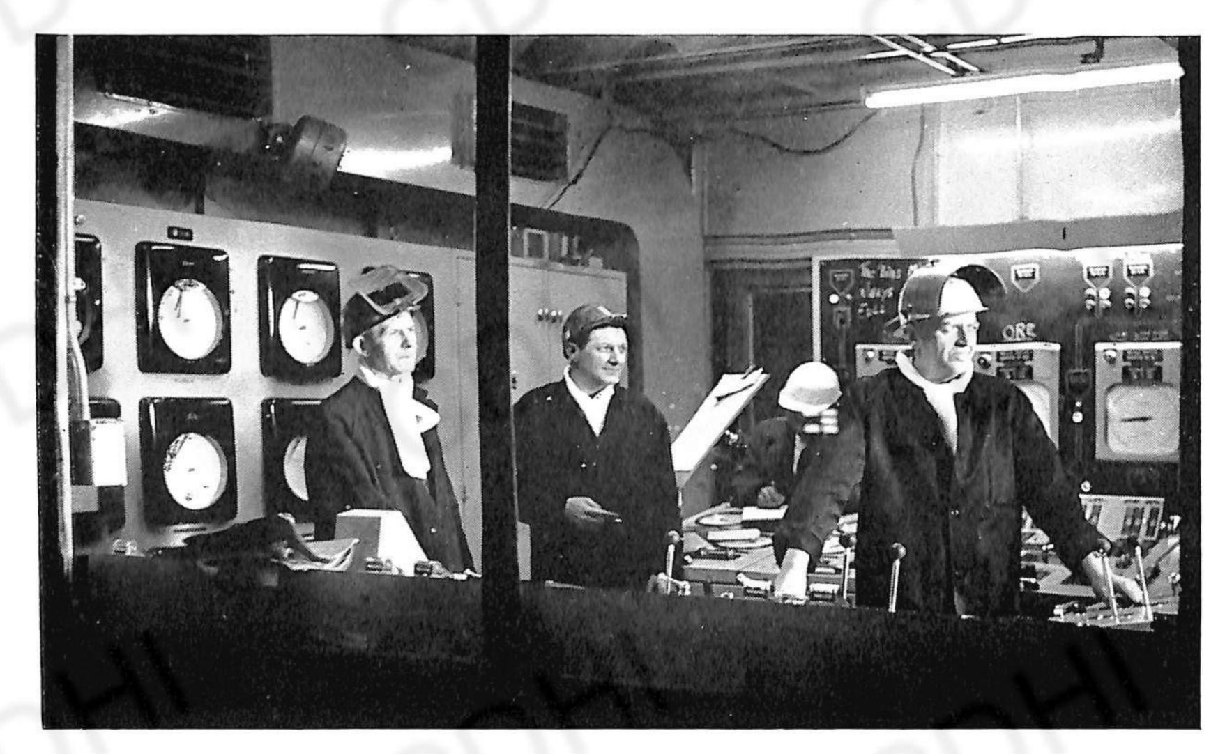
Fig. 6. One of the control pulpits for the Kaldo converter
