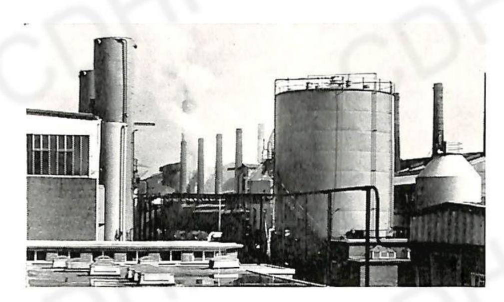
were installed to ensure continuity of oxygen supply — a vital factor in the pneumatic steelmaking processes. As a further "back-up", liquid oxygen storage of 21 million ft³, or 800 tons, was also provided.
